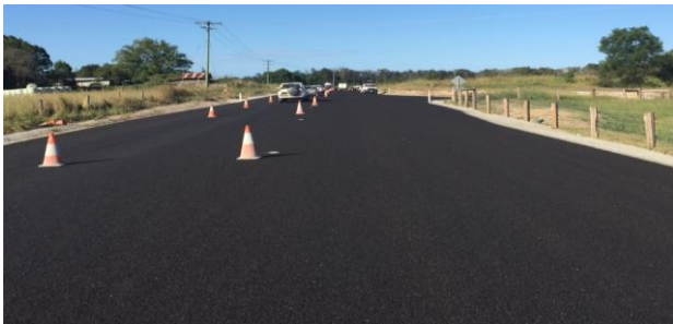
Nearing completion at Sweedmans Lane, May 2016
